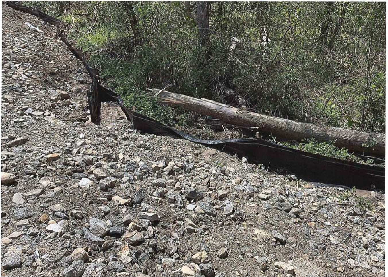
PHASE 4B - SILT FENCES
