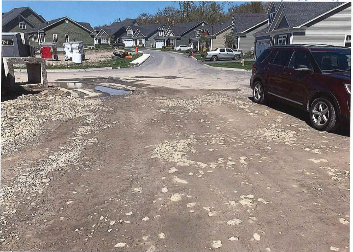
PHASE 4 C - ANTI-TRACKING PAD / Pavement
