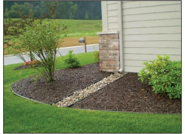
Gutter downspout discharging to lawn.
