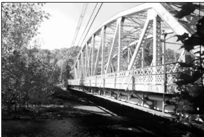
South truss section of the 212 foot long, Depot Street Bridge as viewed from the east bank of the Naugatuck River, circa 1940. The bridge, built in 1934 to replace an existing wooden bridge, is an example of Parker truss Design.
